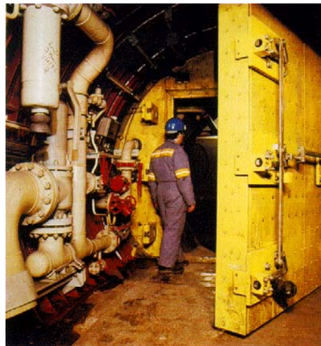
Above, left: Pumping station « K », one of 3 undersea. Right: inside view of the French Pumping station « W3 ». Below, left: One of the 270 Cross-Passages, with door open. Right: one of the 194 Piston Relief Ducts.
