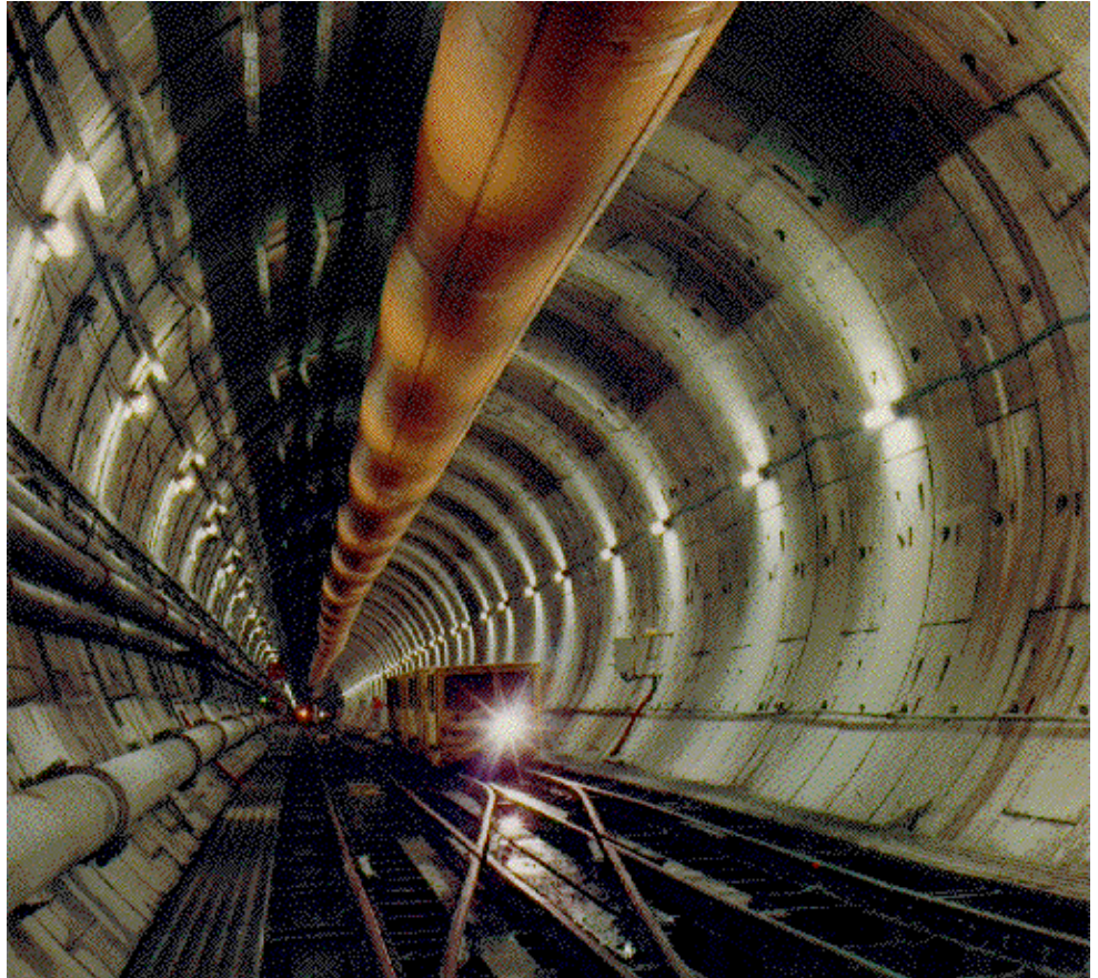
Above : View of a running tunnel on French side at the beginning of the tunneling phase (1988), showing temporary fixed equipments (water pipes, ventilation duct diam 1600mm, power and radio communications cables, double track and walkways...). Below : Tunneling progress on 29th of April 1990, 7 months before first undersea breakthrough, showing forecasted ("M"), and final (black balls) meeting points.
