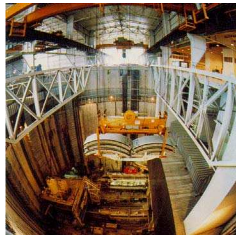
Above: Sangatte Shaft (55 m diam, 65 m deep), concentrating all tunneling activities on French side. Below : View inside the shaft. 6 precast segments are being transferred into tunnels.
