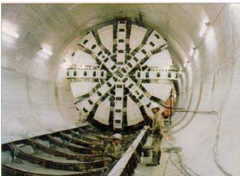
Above : Launching the "T2" Tunnel Boring Machine (TBM) from Sangatte Shaft (running tunnel north undersea). Below : Inside the control cab of a TBM.
