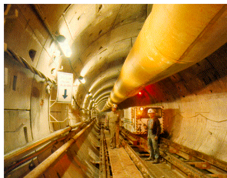
Tunnel views during works, showing temporary equipments (trains, track, water pipes, power and communication cables..): Service Tunnel (above) before breakthrough with ventilation duct. Running Tunnel (below), near a piston relief duct, with still temporary catenary, track, and pipes, but also some of the permanent equipment already installed.
