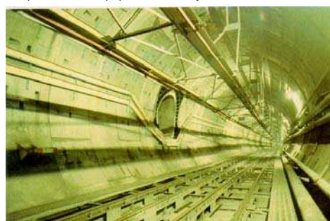
Tunnel views during works, showing temporary equipments (trains, track, water pipes, power and communication cables..): Service Tunnel (above) before breakthrough with ventilation duct. Running Tunnel (below), near a piston relief duct, with still temporary catenary, track, and pipes, but also some of the permanent equipment already installed.
