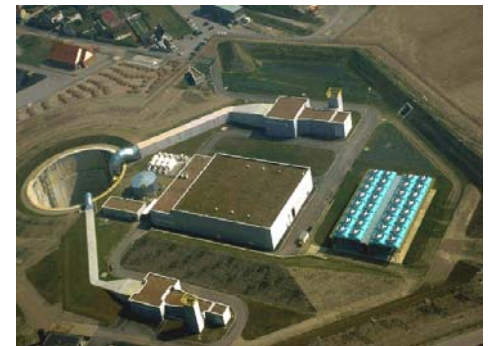
Sangatte Shaft today : The Shaft is not covered any more. Inside, technical rooms, reconstituted tunnels, and ventilation ducts have replaced the former, complex tunnelling logistics. On surface, permanent facilities (cooling, ventilation, fire fighting, diesel power plant) have replaced, in a now landscaped area, the huge construction facilities.
